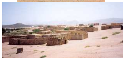
Rural decentralised electrification in Algeria
